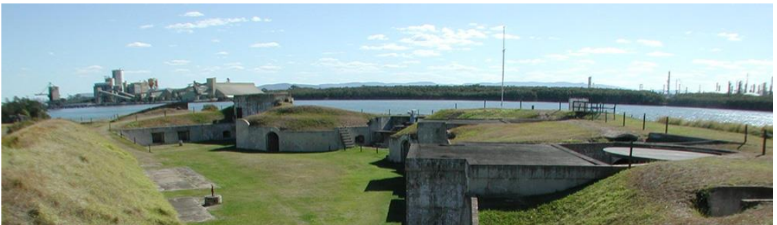
SITE LOOKING TOWARDS BRISBANE RIVER
